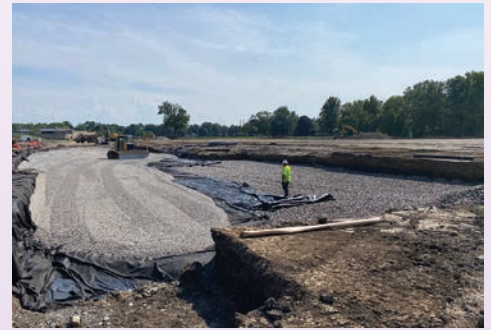
Construction of the stone subbase at the new bus loop
