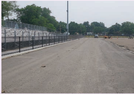
New fencing and sidewalks at Howe Field
